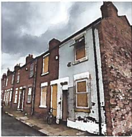
Abandoned terraced housing in Doncaster
